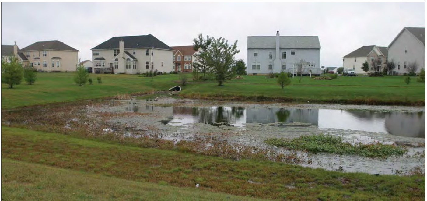
The increase in stormwater ponds, while important for surface water detention, are no substitute for the multitude of functions provided by natural wetlands (classifications: palustrine unconsolidated bottom wetland semipermanently flooded and terrene pond isolated wetland; Rebecca Rothweiler, DNREC WMAP )
