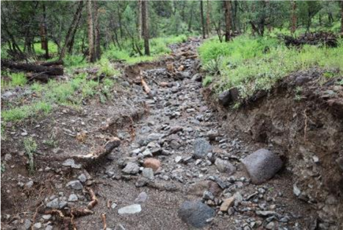
A large log drop that is reinforced with rock to aggrade an incised channel
