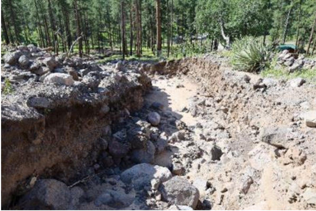
Another sediment catchment in a drainage to the creek
