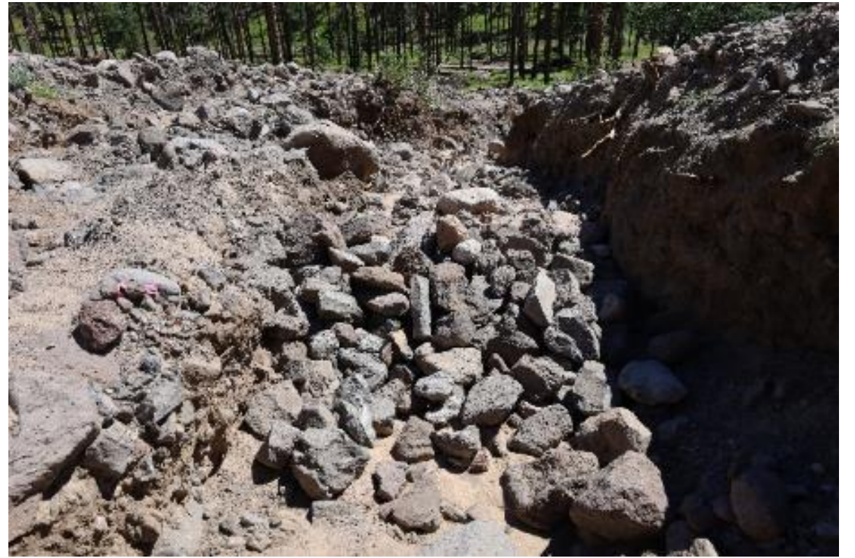
Another sediment catchment in a drainage to the creek
