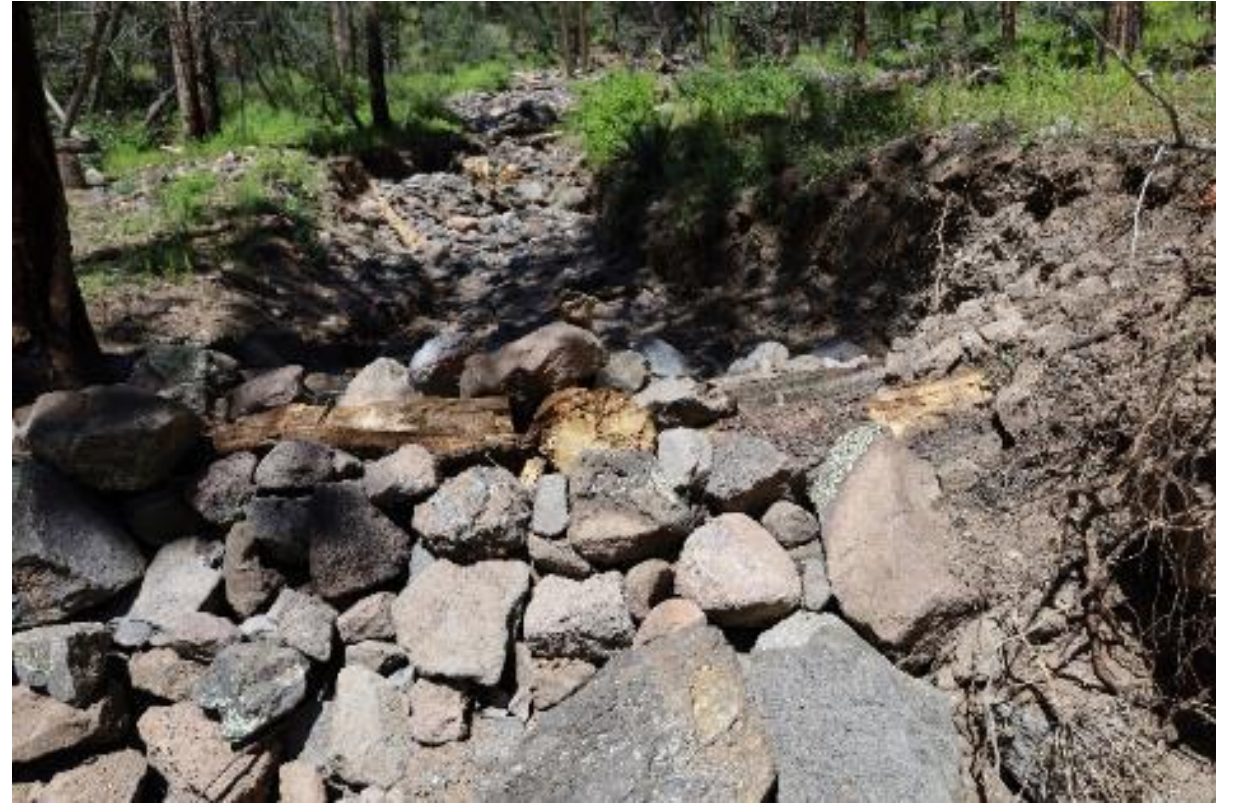
A large log drop that is reinforced with rock to aggrade an incised channel
