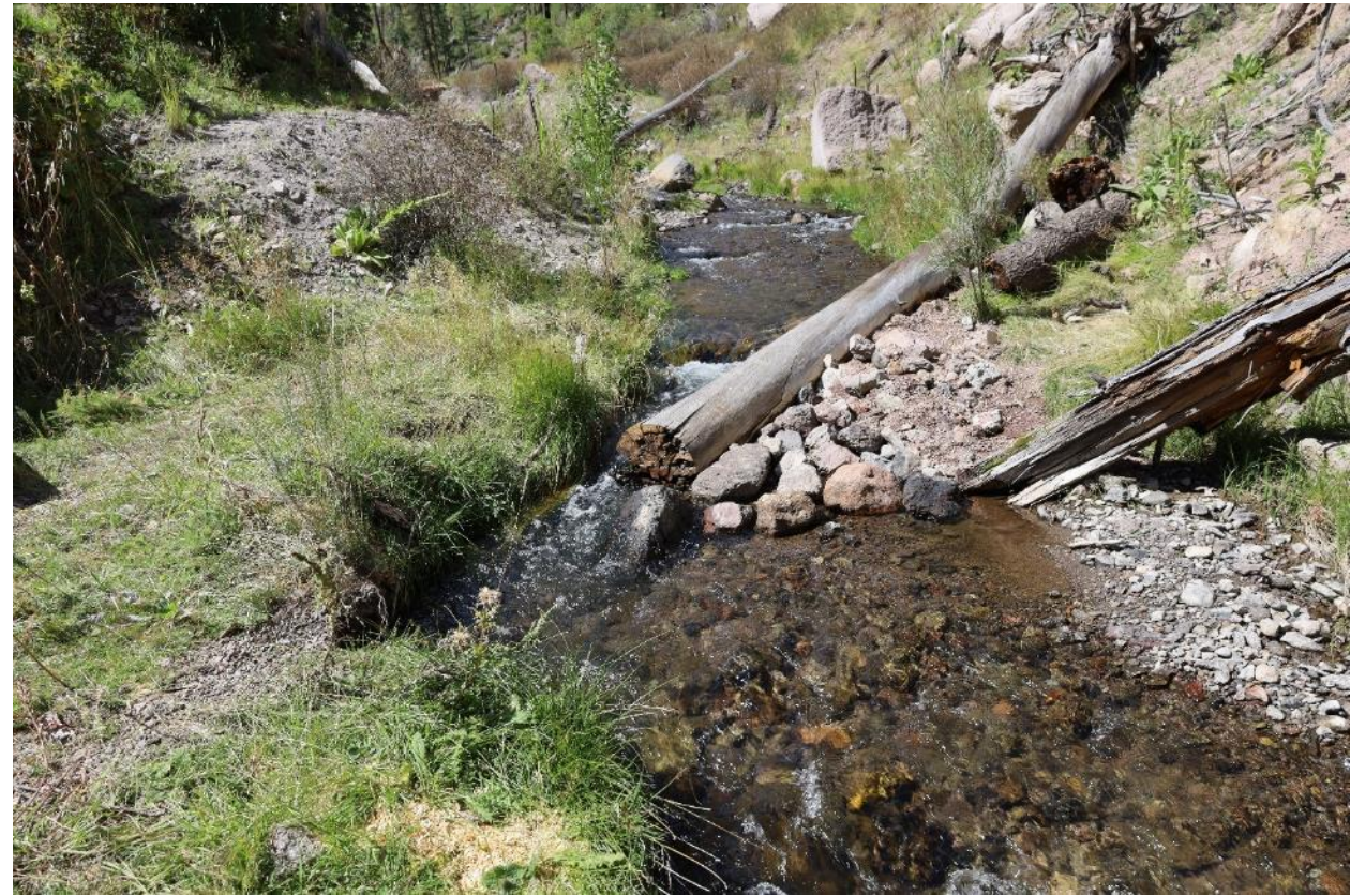
A rock baffle induces a stream meander and adds sinuosity to Santa Clara Creek
