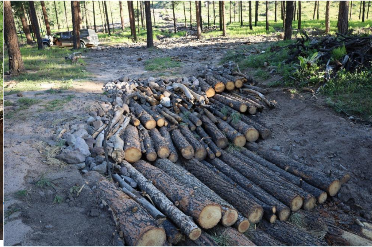
large rundown comprised of logs, rocks and branches placed in severely impacted erosion channel
