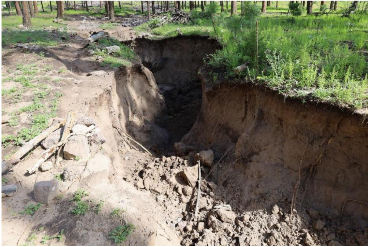
large rundown comprised of logs, rocks and branches placed in severely impacted erosion channel
