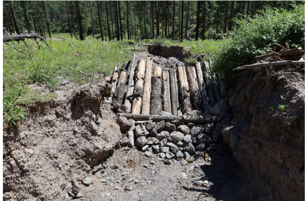
A well-constructed sediment catchment in Santa Clara Canyon
