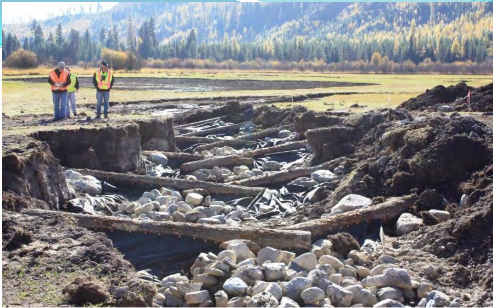
Log Drop Structures being constructed at Schrieber Creek. Note geotextile fabric tacked to upstream end of logs.
