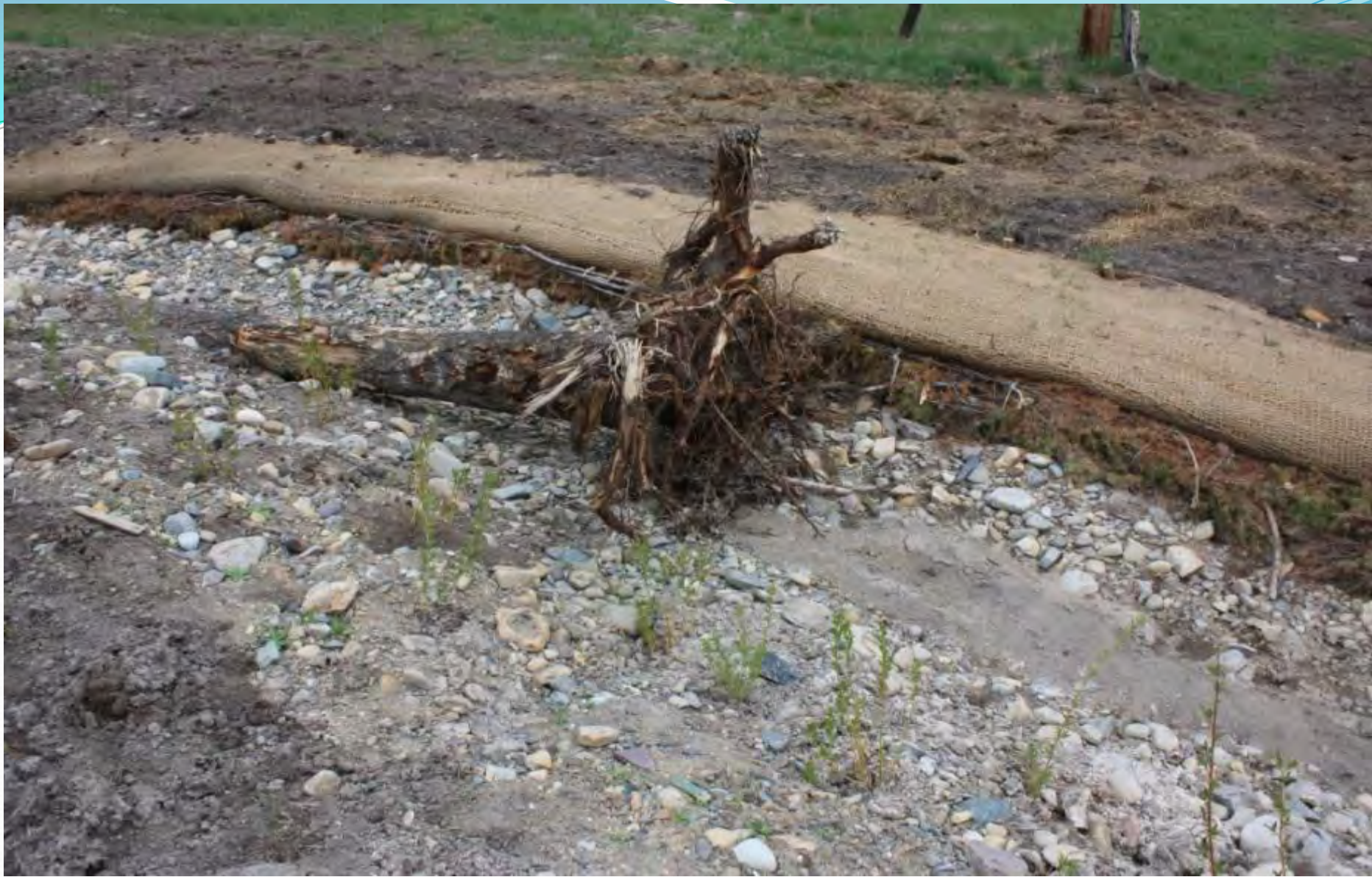
Coir fabric bank treatment underlain by evergreen/willow branch fascines. Note passive wood root wad in stream channel to create habitat and sediment deposition. Woody plantings have been made in point bar location at edge of channel.
