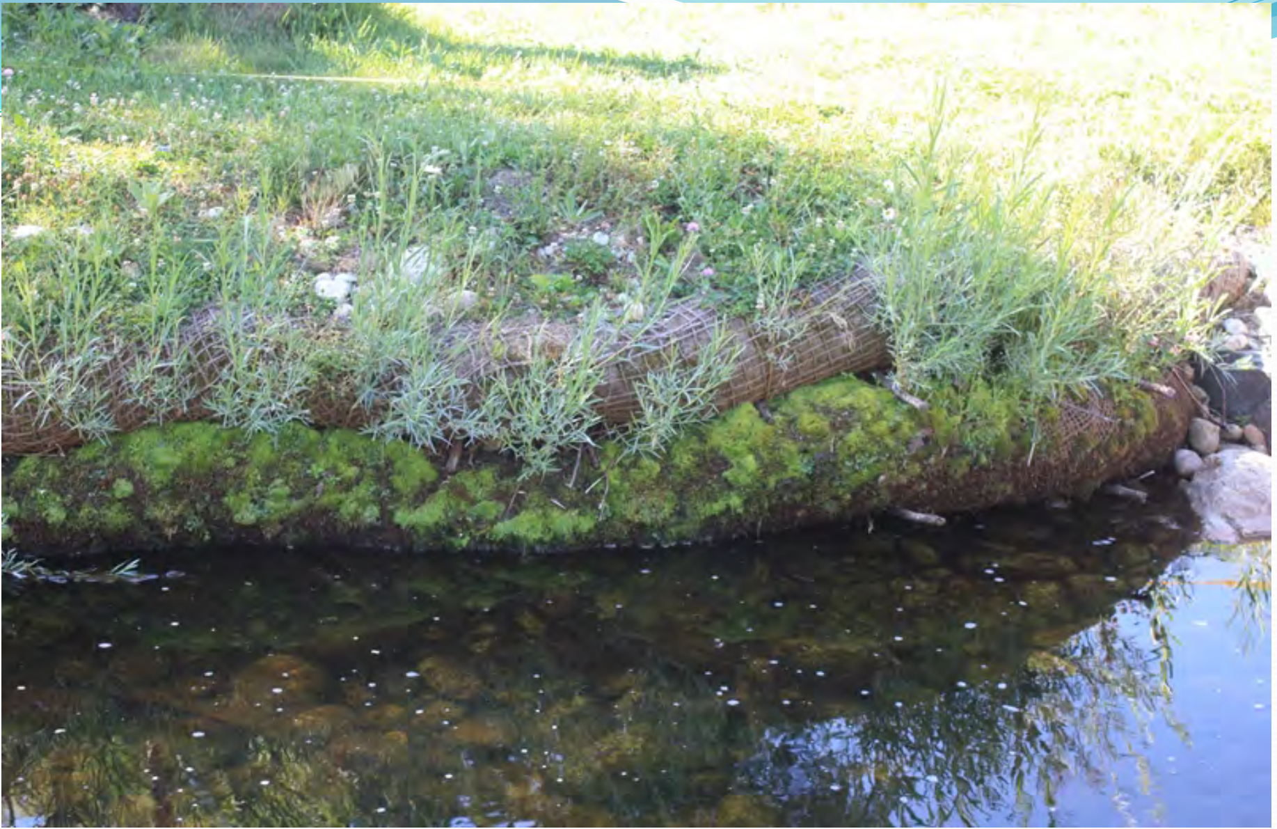
Two coir log bank installation with a rock toe and willow cutting mat between coir logs sprigged with willow cuttings.
