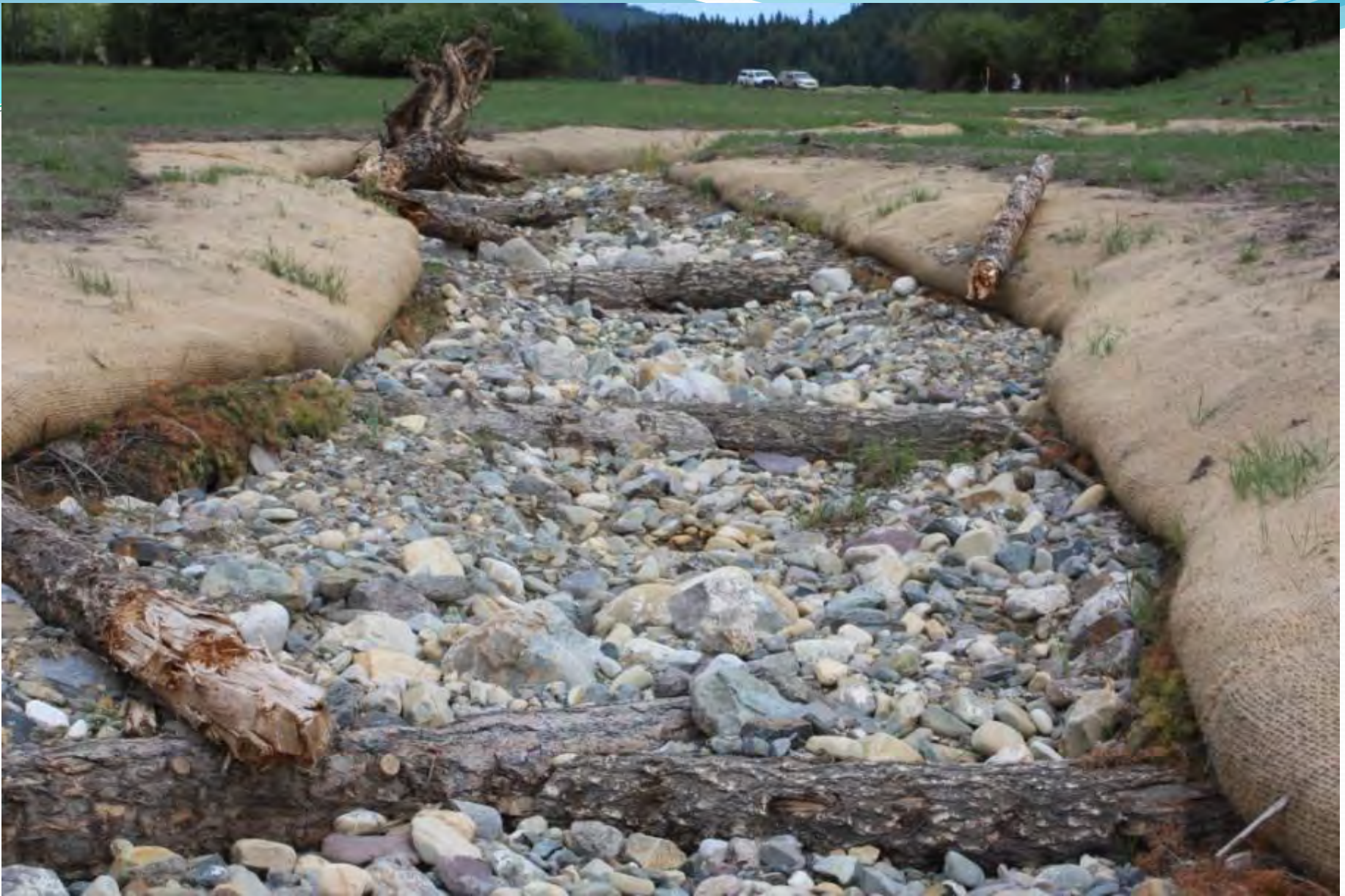
Completed log drop pool structures with coir fabric wrap and fascines on Schrieber Creek channel. Note flat floodplain areas and passive wood.
