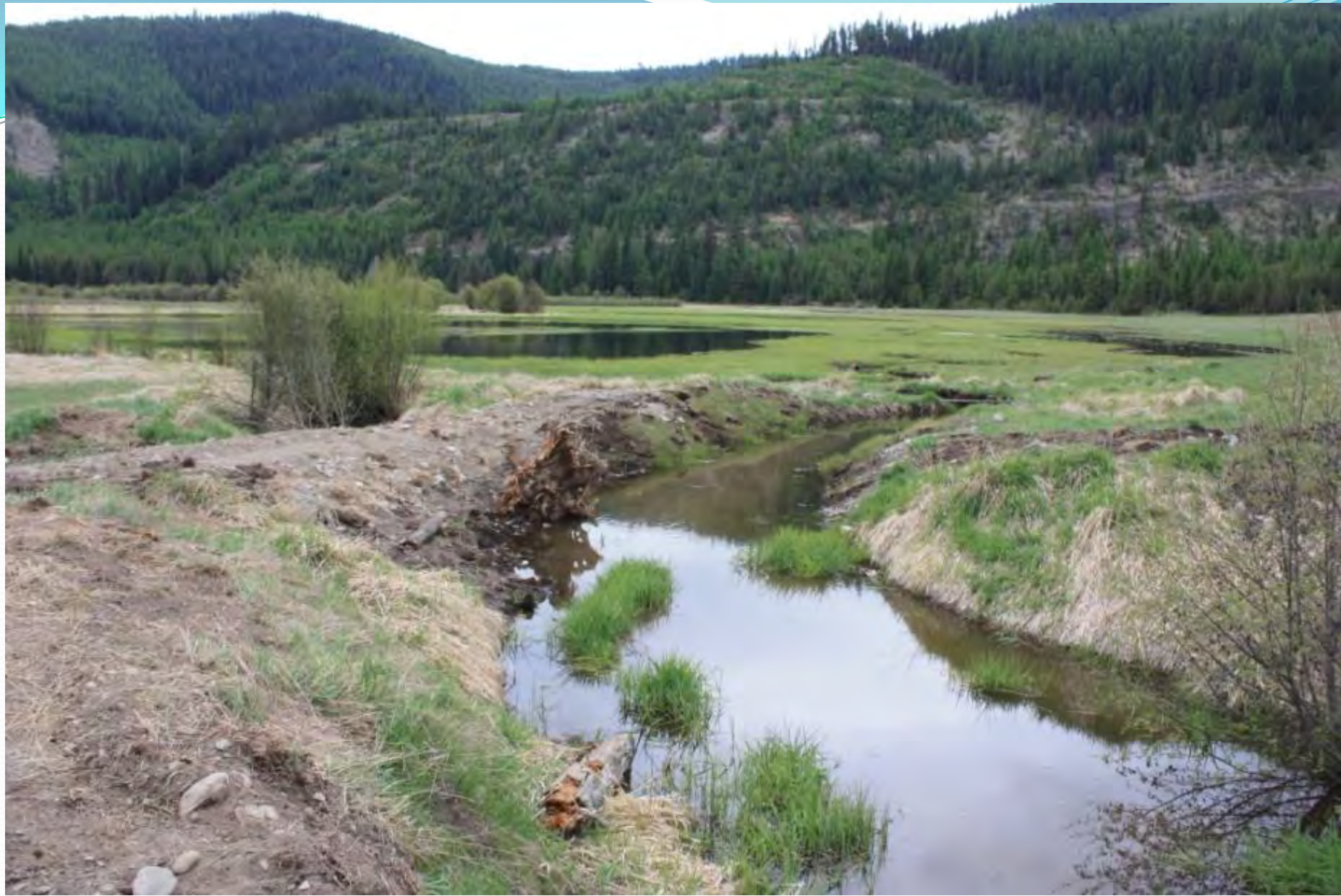
Coyote Creek channel plug diverting stream into new channel. May 2015
