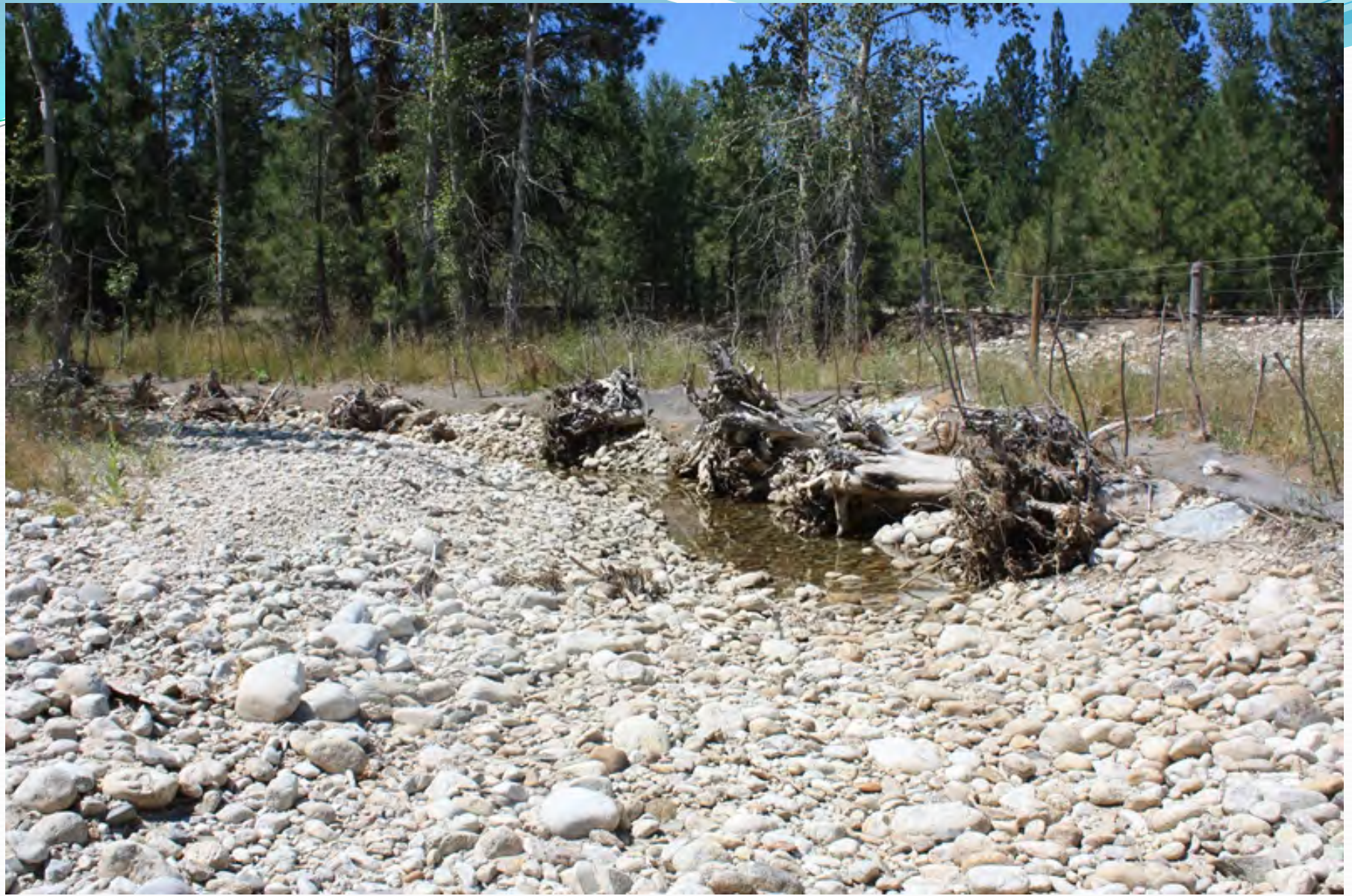
Series of root wad bank structures to serve as flow deflectors and habitat structures in an ephemeral stream channel.
