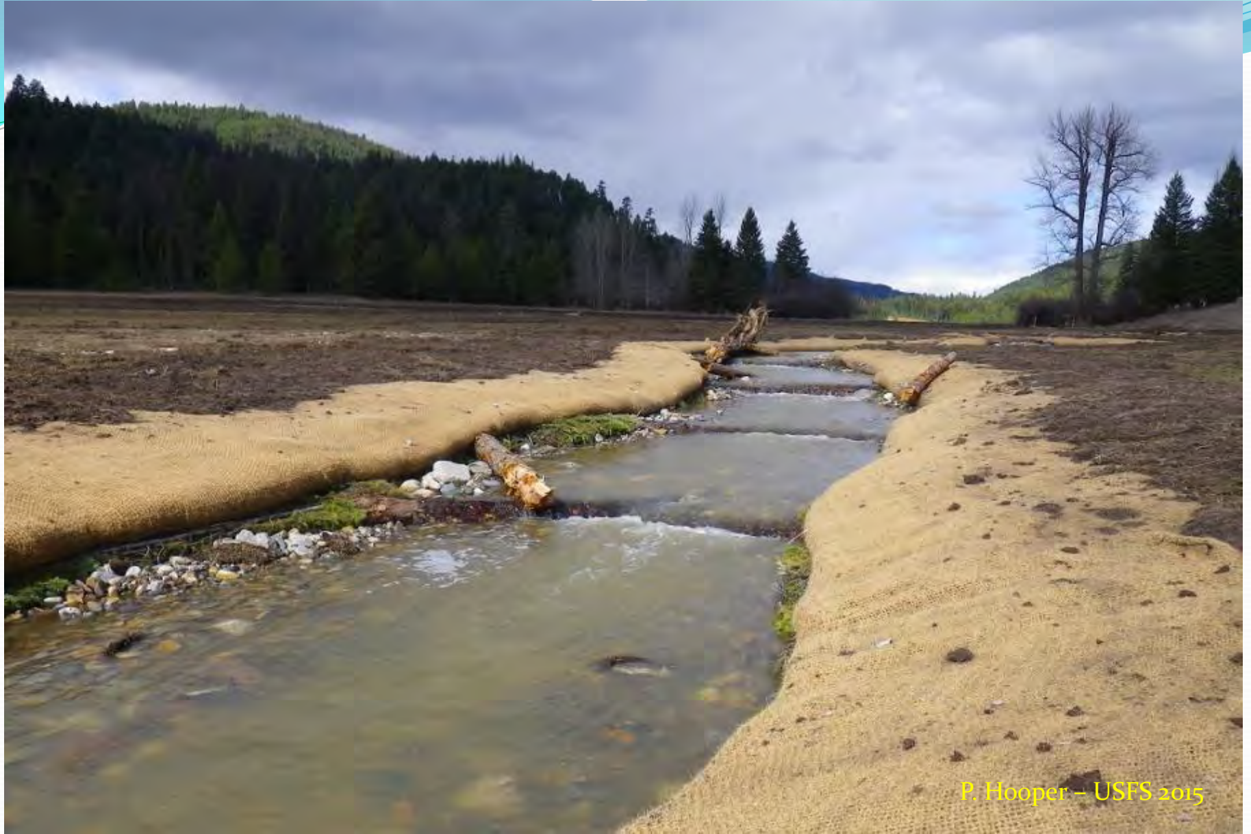
Completed log drop pool structures functioning during spring runoff March 2015.
