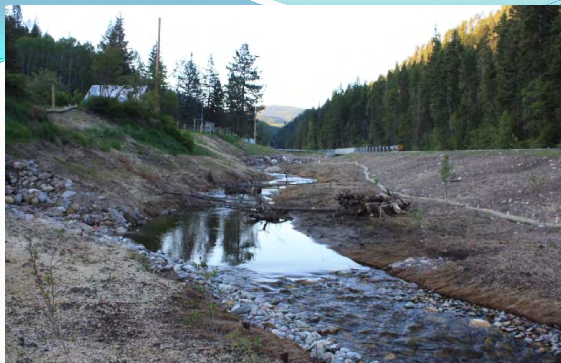
Placement of passive wood in a newly constructed stream channel and floodplain.
