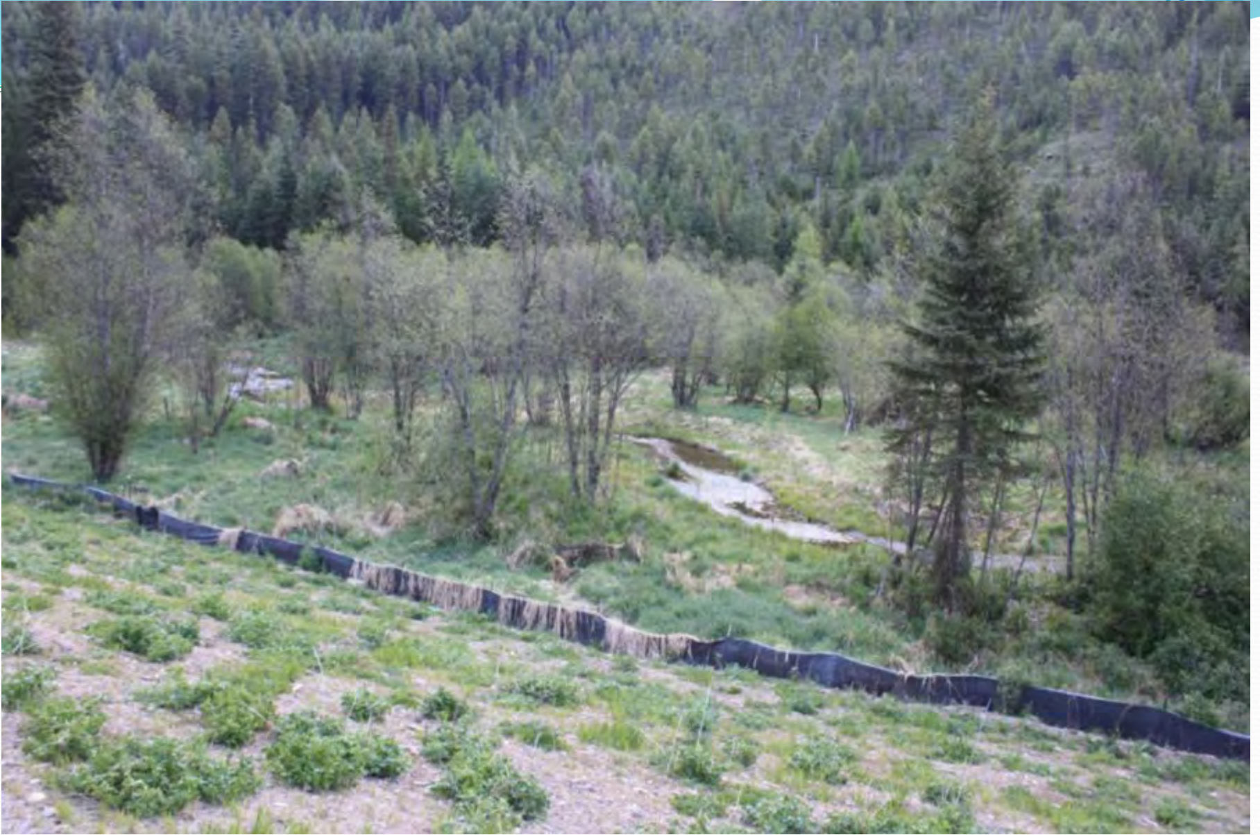
Placement of new channel to naturally fit into the landscape.
