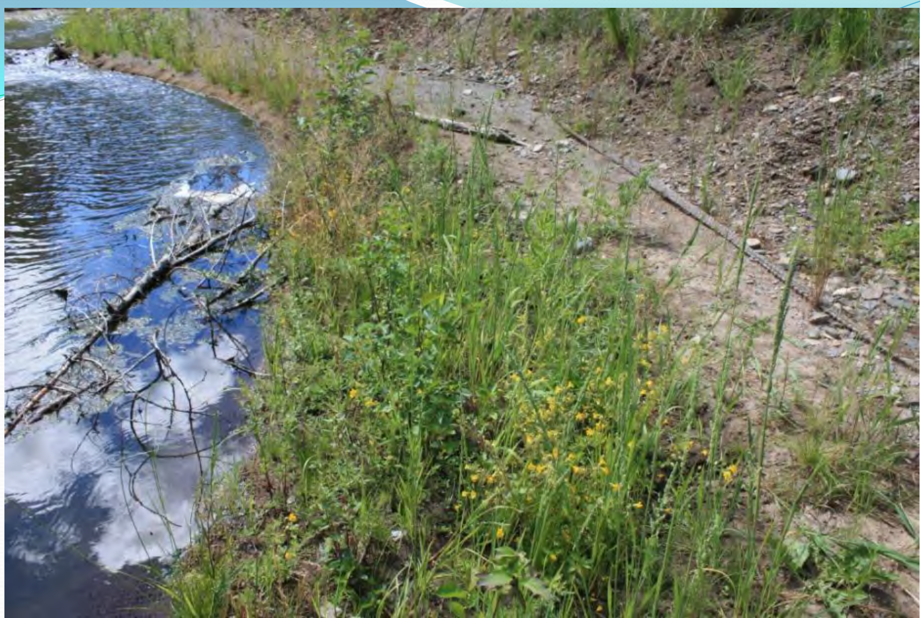
Natural vegetation establishment and sediment deposition on coir fabric streambank wrap within floodplain. Note passive wood in channel.
