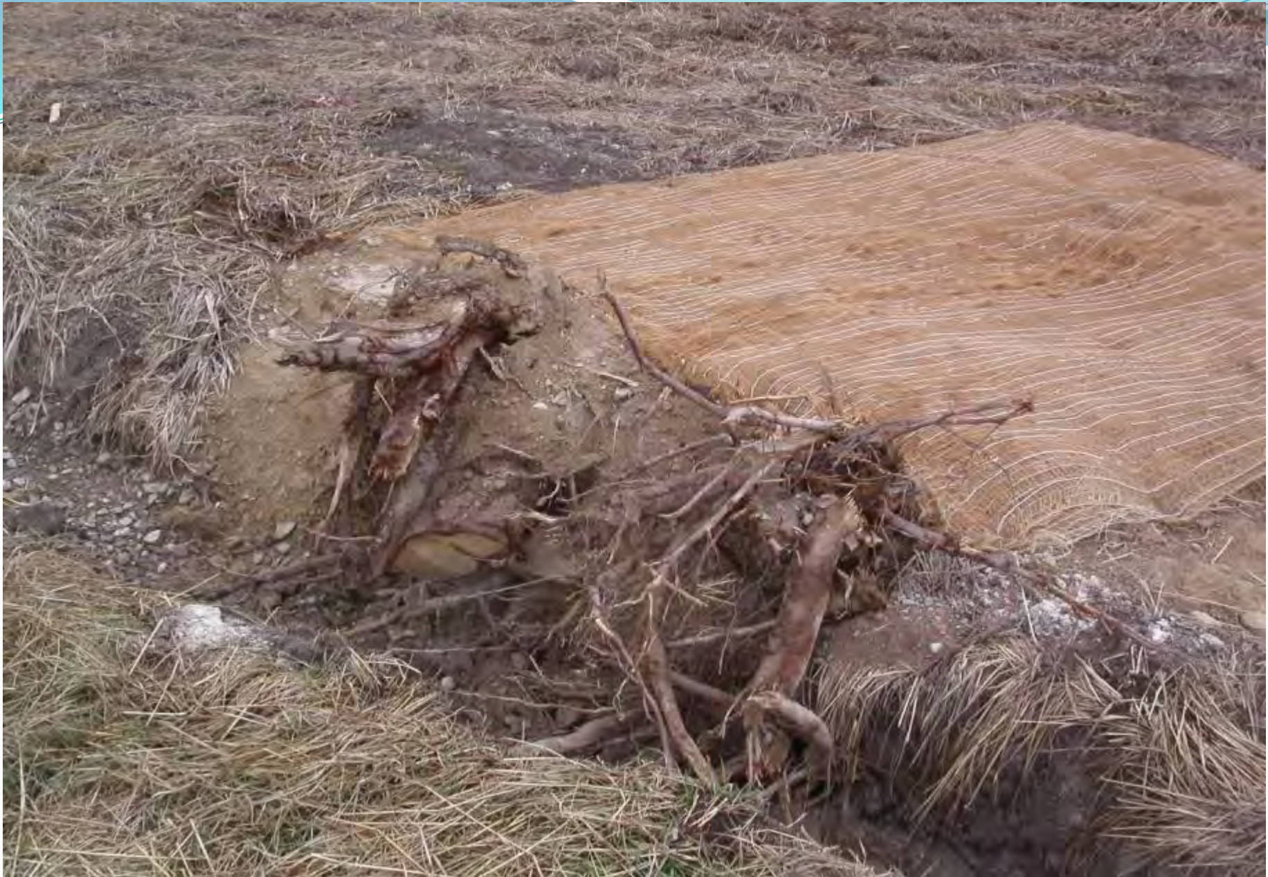
Root wad ditch block installation at Schrieber Meadows – September 2011
