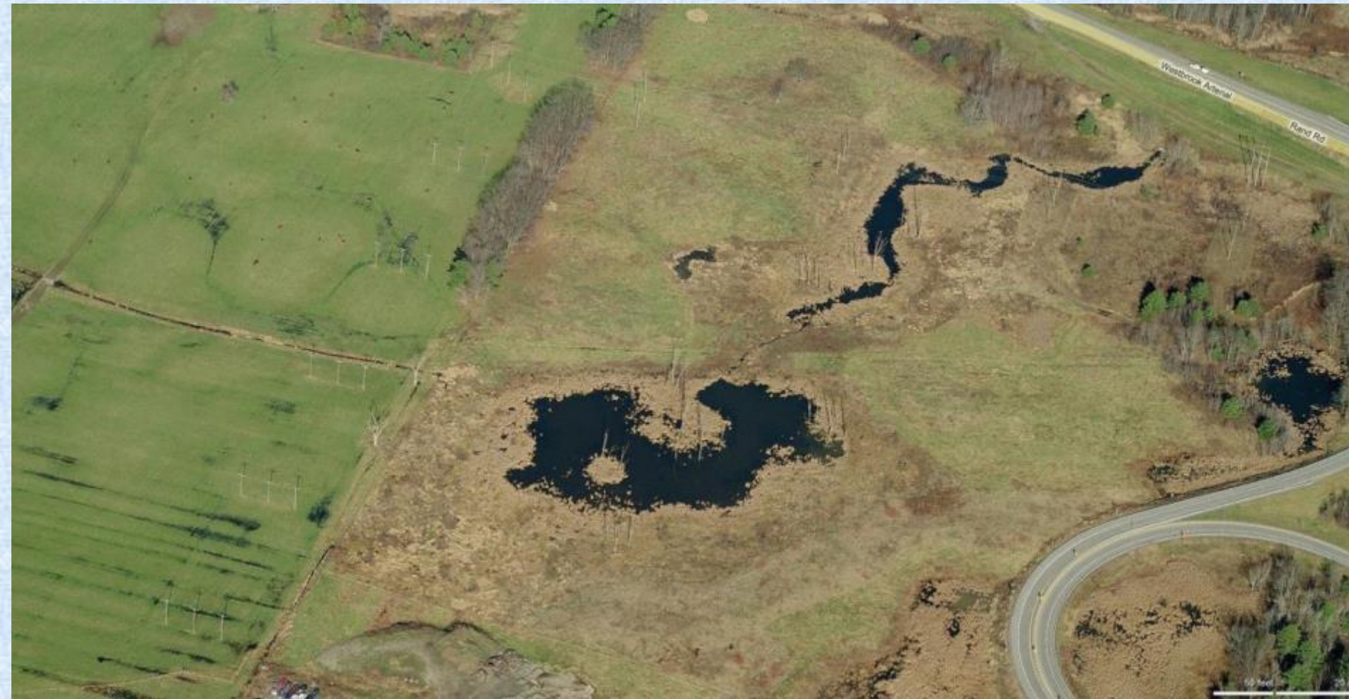
Rand Road Interchange Wetland Mitigation Site, Maine Turnpike Authority
