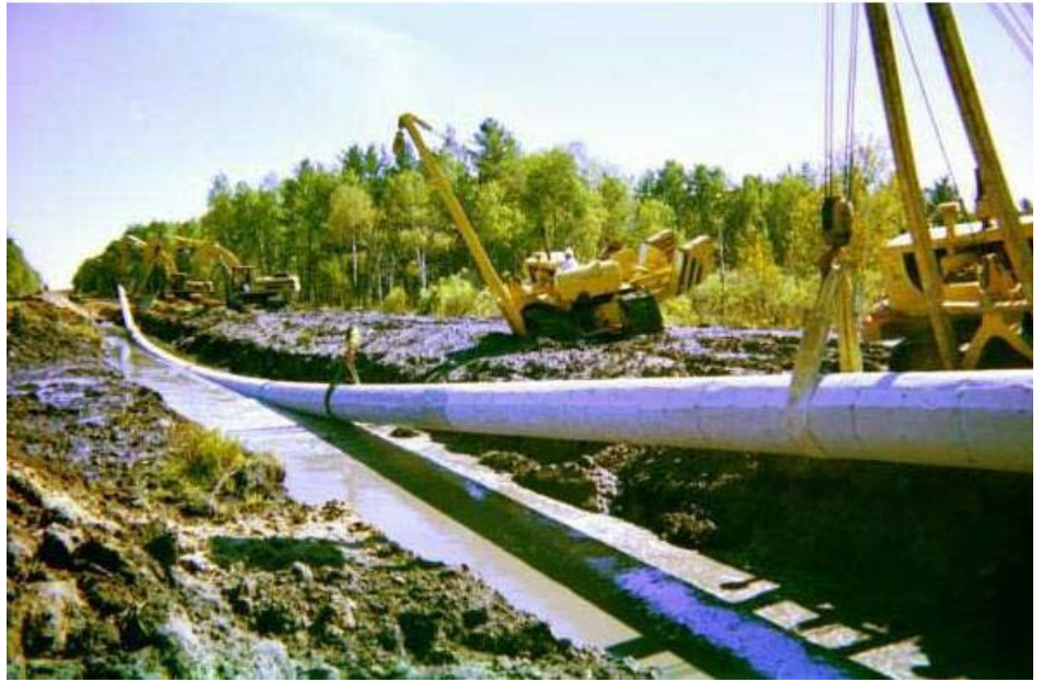
Lowering a Pipe with a Sideboom Photo Credit: Federal Energy Regulatory Commission
