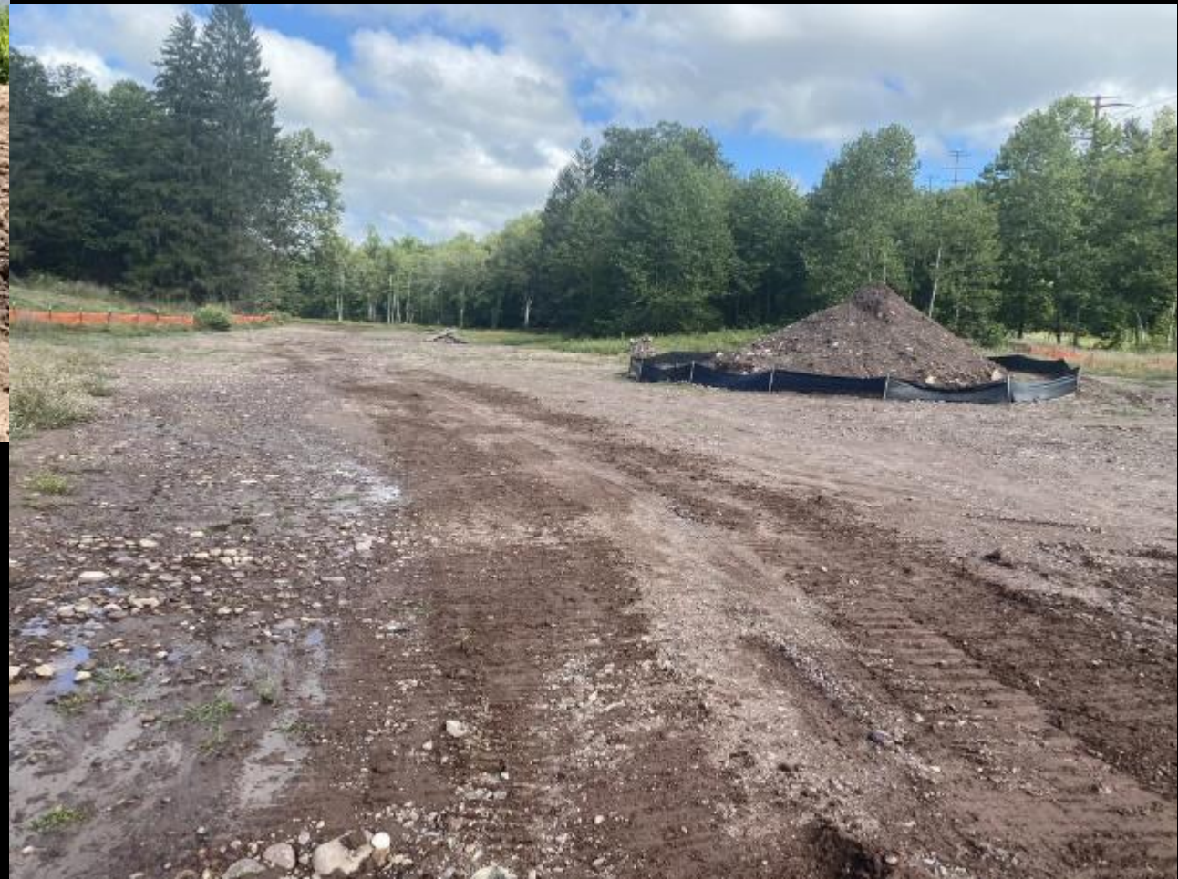
Topsoil Removal & Salvage
