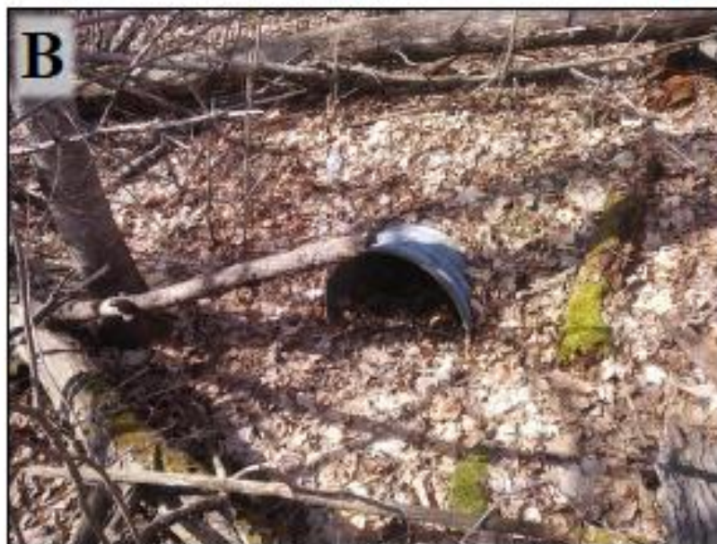
Plate 3. Example jurisdictional break evaluation depicting A) a roadway culvert that exhibits characteristics of at least seasonal surficial flow (ordinary high water marks (OHWM), vegetation preclusion, scour, etc.), and B) a roadway culvert that does not exhibit characteristics of at least seasonal surficial flow. Photos taken by LLBO staff in April 2020.
