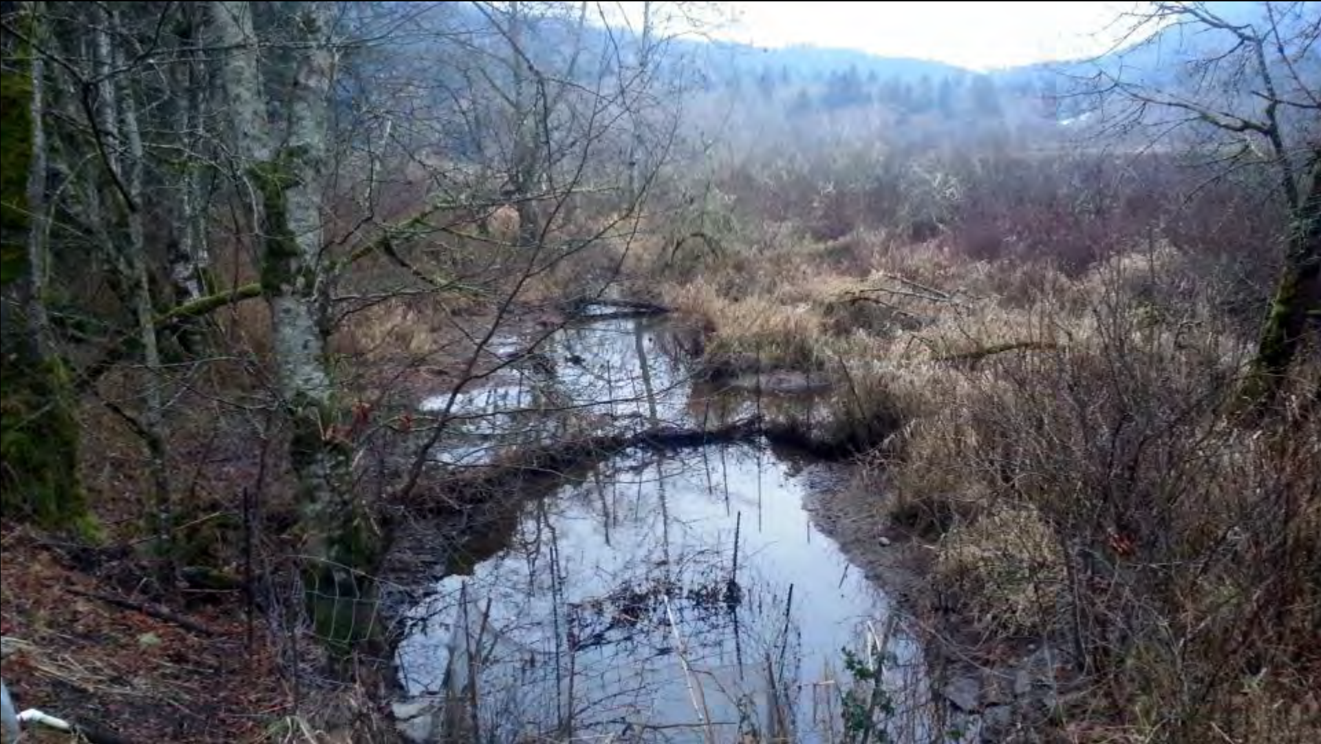
Beaver dam blocking diversion ditch
