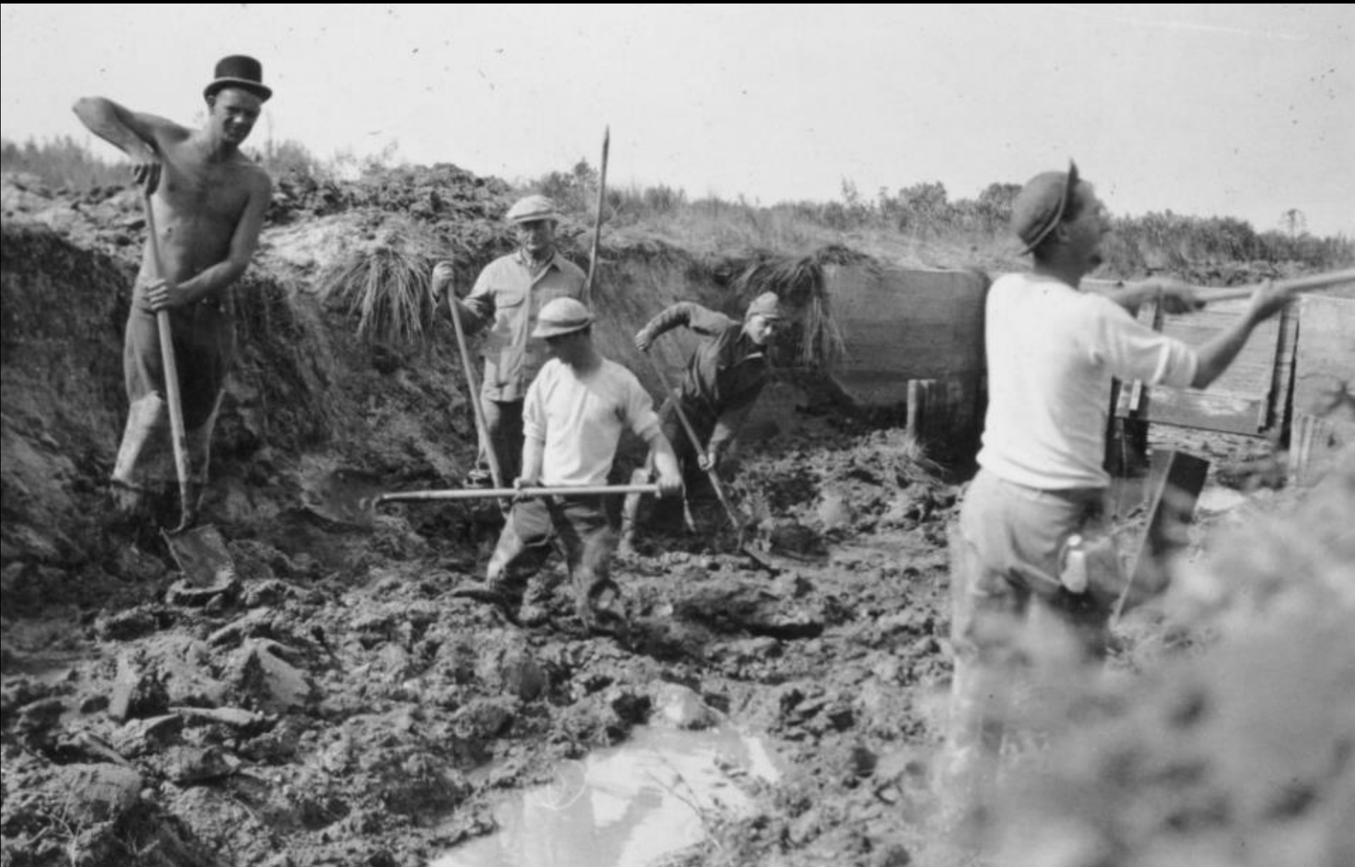
Primehook Creek, Delaware-widening main ditch near the bay
