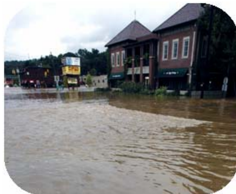
Building in a wetland may result in landowner liability
